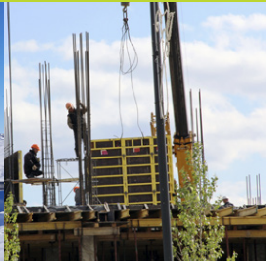
New construction in Astana (Kazakhstan) Photo: Shynar Jetpissova/World Bank
