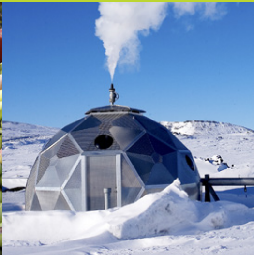
Geothermal borehole house (Iceland) Photo: Lydur Skulason
